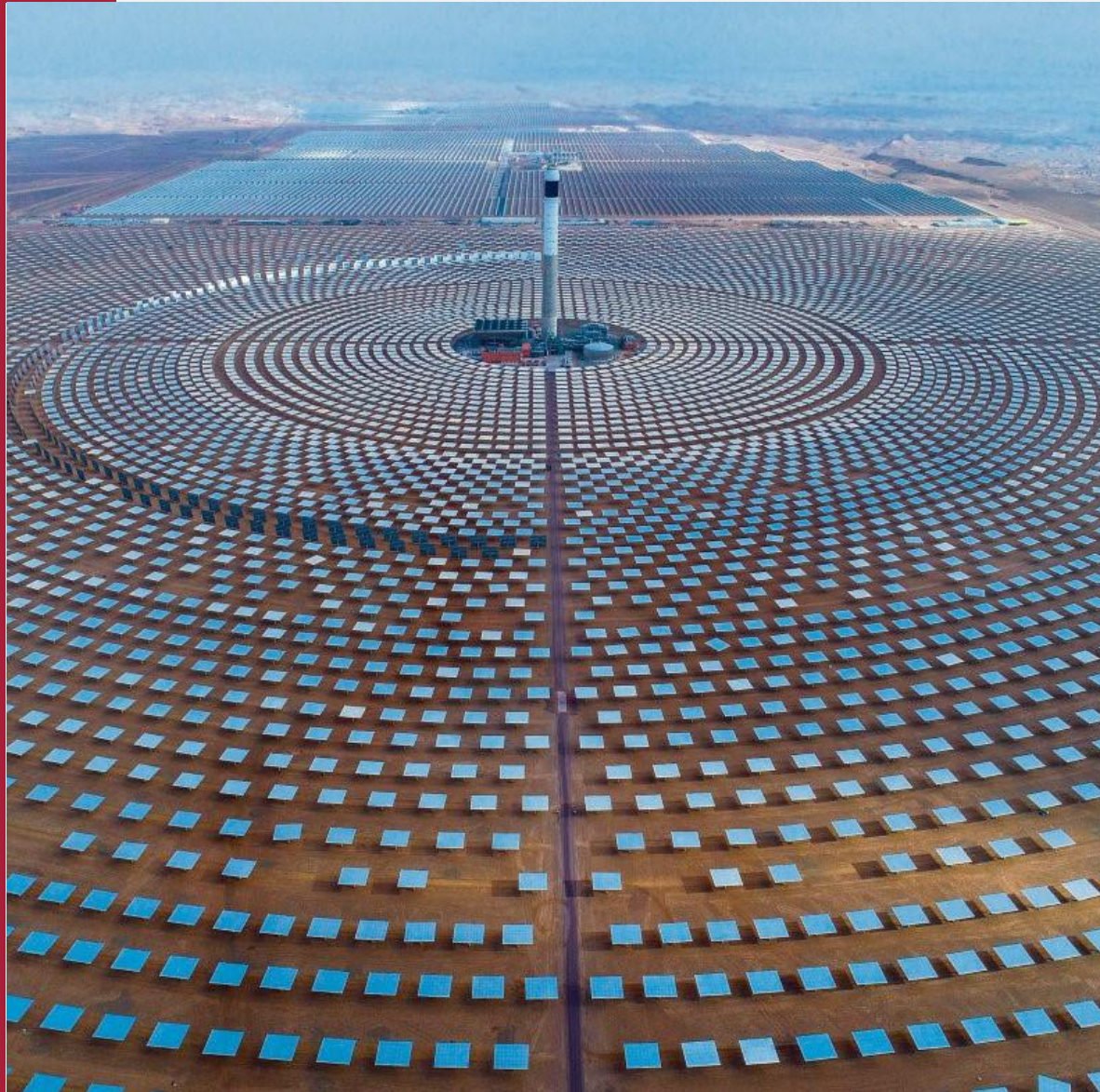
Solar power plant / Noor
